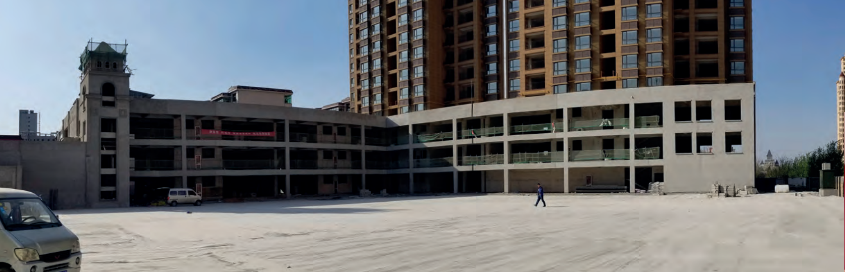
Original site of the Lingbao Children's Center.
