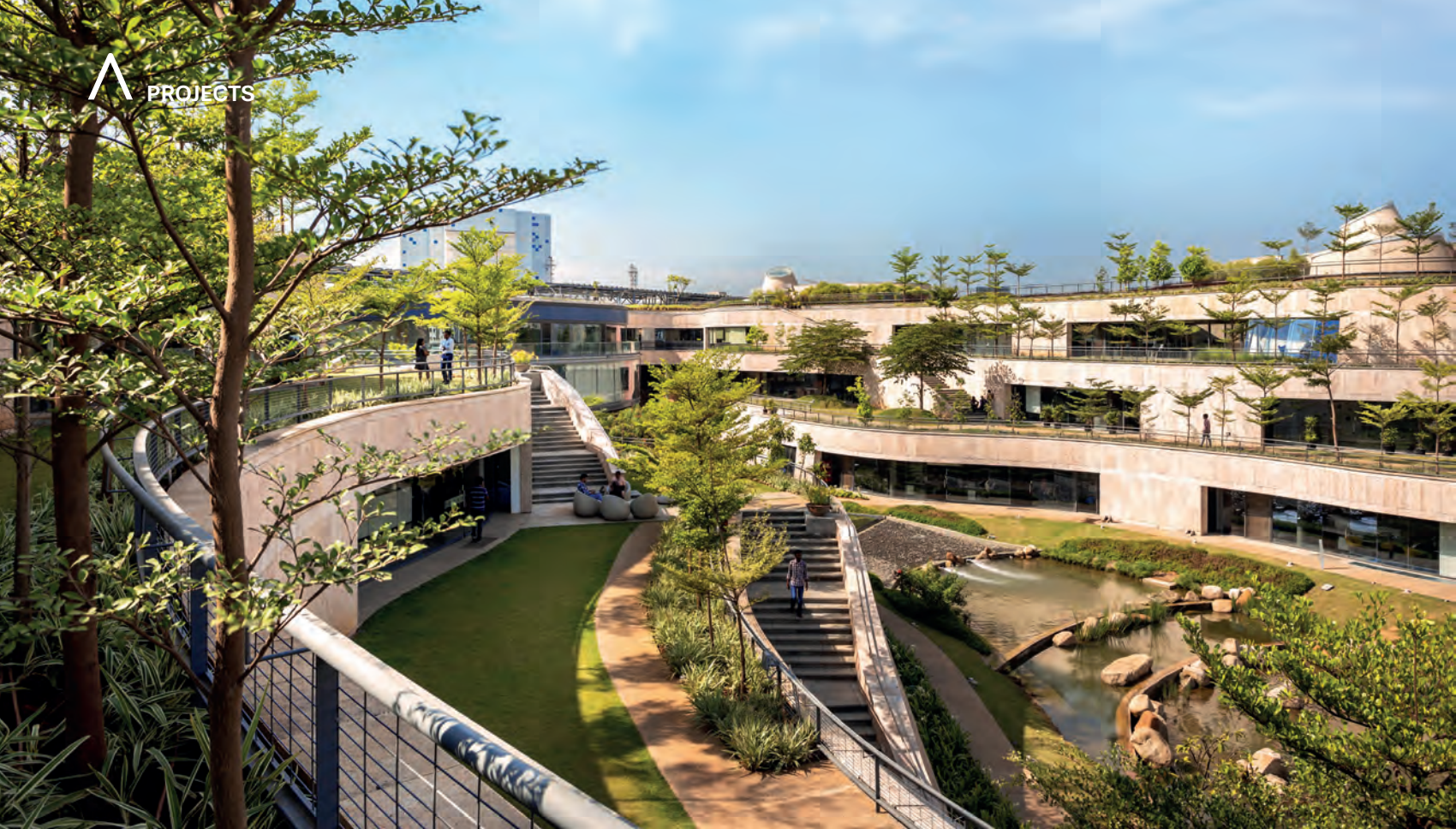
The cascading green terraces along with the lake create an adequate micro-climate thus minimizing mechanical cooling.
