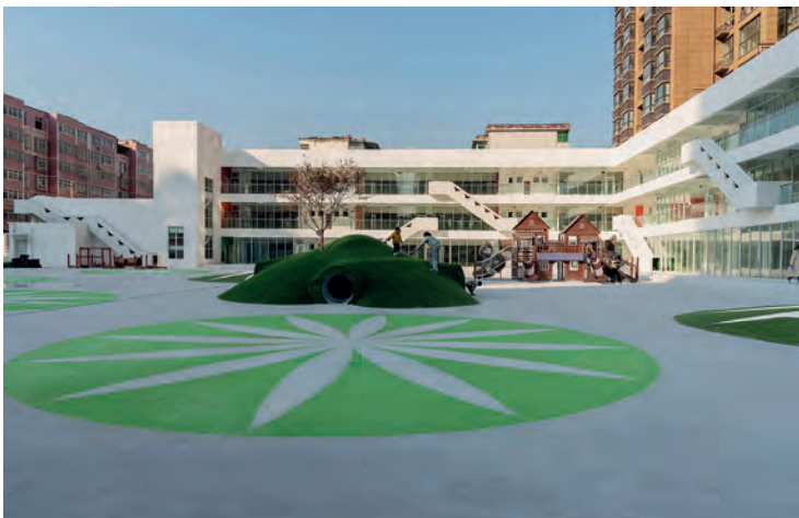
The slides on the building and the hillocks on the playground create happy undulations.
