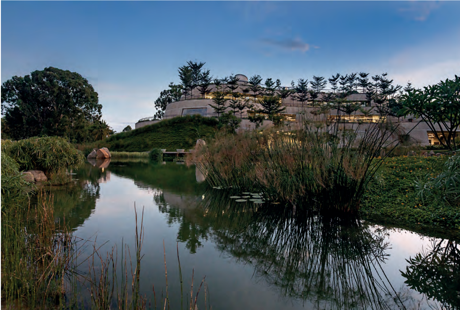
The Lake does not only act as water retention, but also acts as a secondary fire storage tank in case of emergency.
