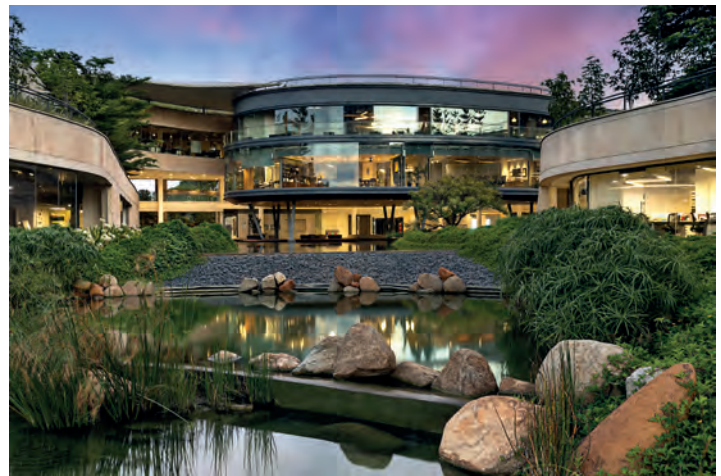
Bio Lake helps to increase wildlife footprint within the city and integrate the design well with the surrounding.
